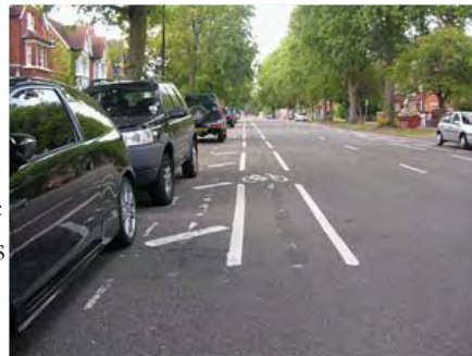
(Top) An example of a bike lane located within the “door zone” of the adjacent parallel parking lane. (Bottom) Providing a striped buffer between on-street parking and a bicycle lane is a potential design solution to encourage riding outside the “door zone”.
