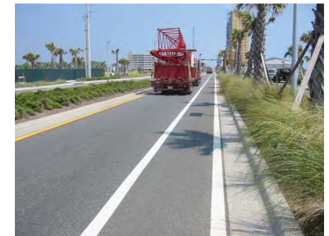
This road in Panama City Beach, FL has 10-foot lanes (which easily accommodate large trucks) adjacent to 5-foot designated bike lanes (4 feet of asphalt, plus gutter pan).
